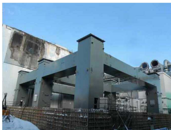
The first layer of steel framing completed
