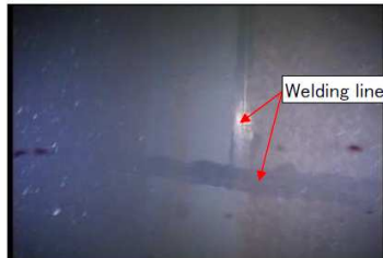
① Southern Wall Surface
